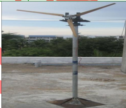
Figure.6 Assembling of Micro wind turbine
