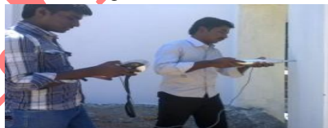
FIG 4.1.Rebound hammer testing of column
